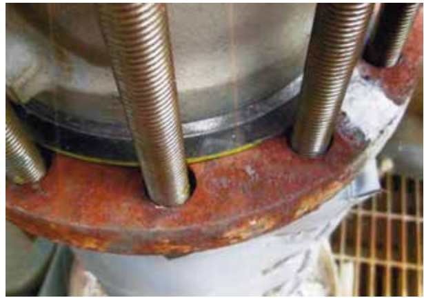
Figure 4. Uncompressed external windings in a wafer valve application.
