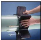
5. Align the buckles and lock into place. Take the final Slide-Lock and slide into place.
