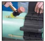
7. To tighten RANGER II® securely to carrier pipe, back Slide-Lock completely out of the slot. If needed, push segments together by hand.
